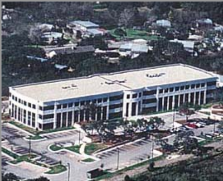
Las Cimas Phase II/III, under construction on S. 360
